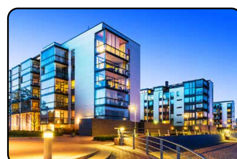
Building Security Control
